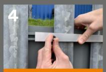
Place the washer under the nut and tighten to hold the panel in place
