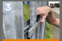
Position the flat bar over the bolts on the other side of the fence as shown
