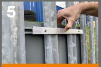
Repeat the process with the bottom run of channel to secure your sign
