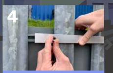
Place the washer under the nut and tighten to hold the panel in place
