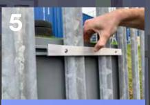
Repeat the process with the bottom run of channel to secure your sign
